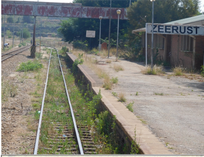
The 'main line', indeed the only line northwards out of South Africa. This line through Zeerust is part of Cecil Rhodes 'Cape to Cairo' line.
