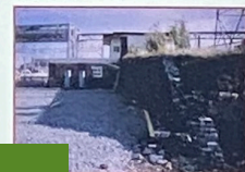
1987 Crewe Works after the Spider Bridge was demolished
