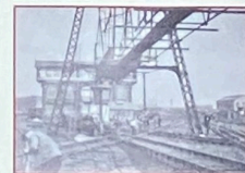
1939 Demolishing the Spider Bridge
