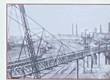
1878 Loading through the Chester Question Box
